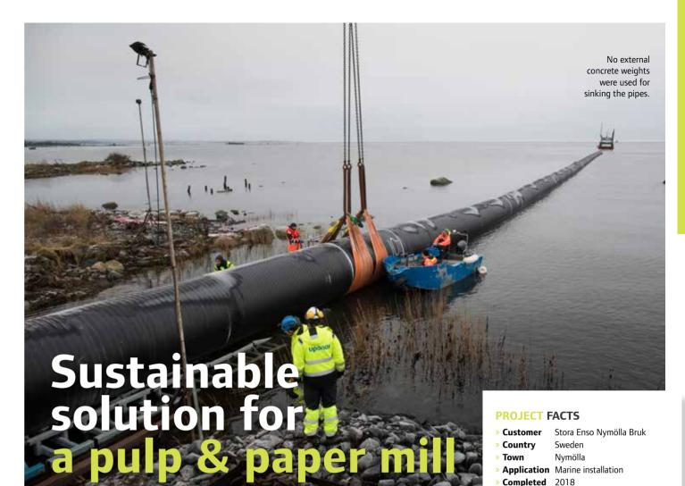
Weholite's ability to withstand external wear, such as friction against the seabed, was an important criterion when the outfall pipe of Stora Enso's pulp and paper mill in Nymölla, southern Sweden, had to be replaced.
