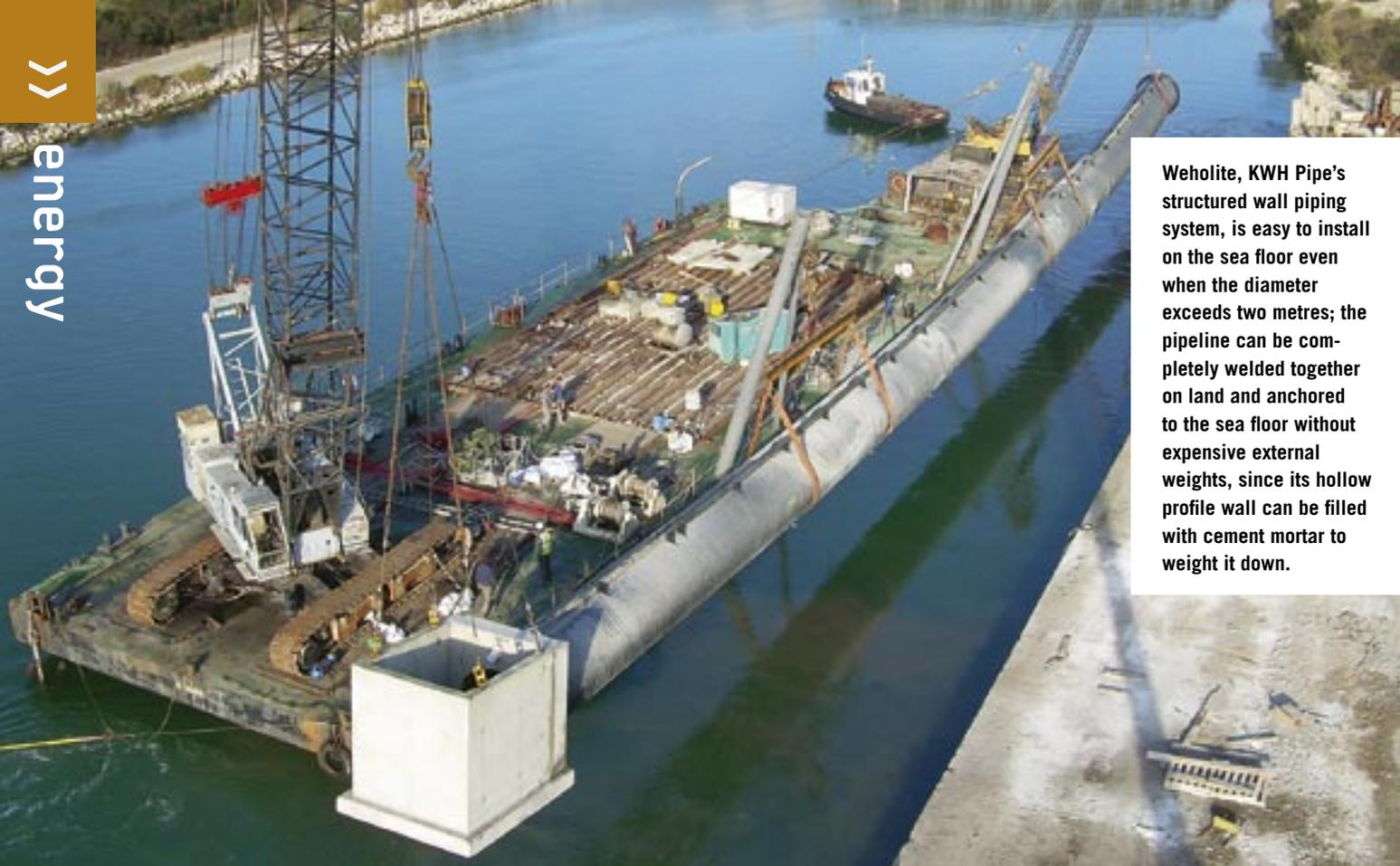
Weholite, KWH Pipe's structured wall piping system, is easy to install on the sea floor even when the diameter exceeds two metres; the pipeline can be completely welded together on land and anchored to the sea floor without expensive external weights, since its hollow profile wall can be filled with cement mortar to weight it down.
