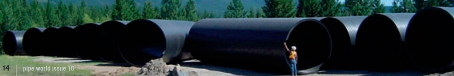
Västerås is building a simple light-weight stormwater pipe system with plastic pipes that are threaded together into long, tight and durable pipelines.
