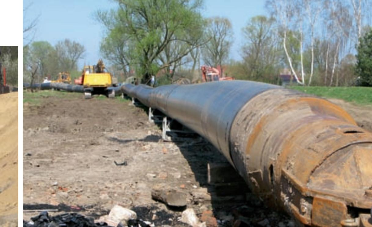
The pipes were pulled over considerable distances. The difficult installation environment and the wish to minimize the burden on the inhabitants were taken into account.
