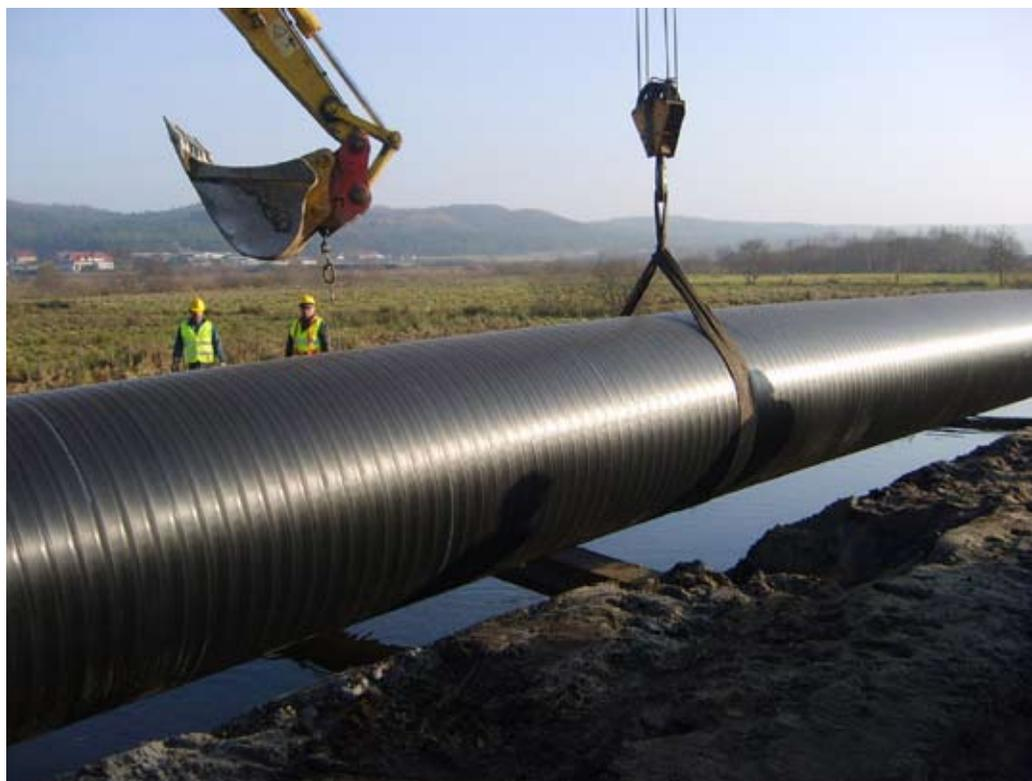
of Kazimierz, while bearing soils comprised the remaining 1 kilometre of the watercourse. Hence, each section required different preparation of the channel bed. The pipeline was founded in bearing soils on a layer of well-compacted gravel whereas the gravel fill layer was additionally wrapped up in geotextile at the weak soil section.
