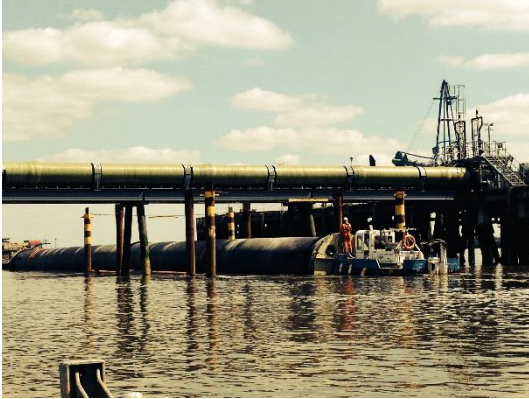
Weholite strings being tugged under the pipe bridge
