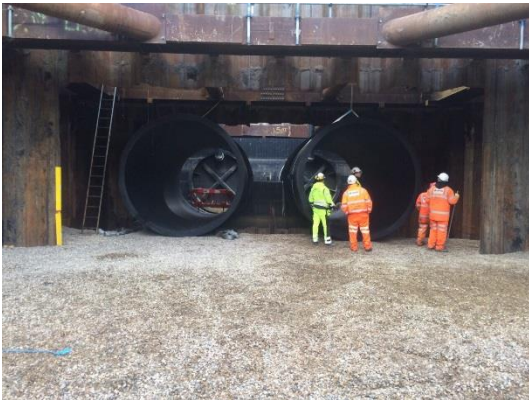
Preparations for connecting to the concrete shaft.
